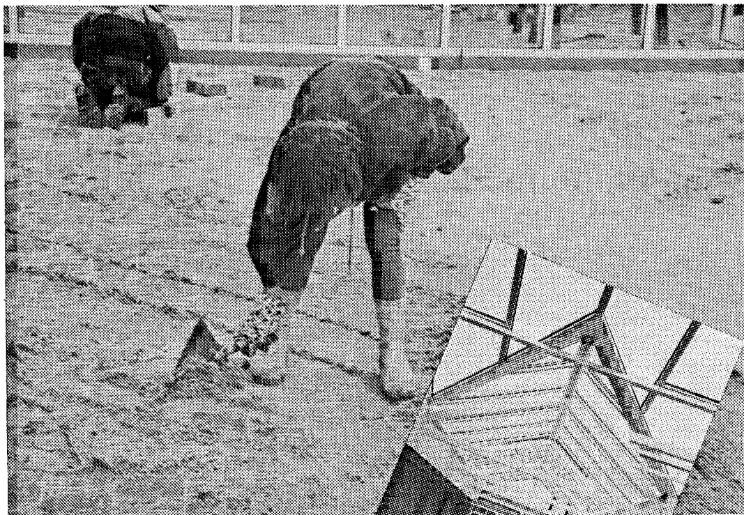
Easter in Klint: children helped to put sand between the new paving stones (left), the new wing (right)
